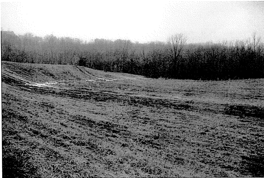
PHOTO 8 – PANORAMA FROM FLOOD WALL LOOKING EAST
