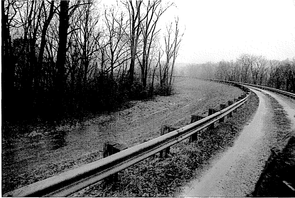
PHOTO 13 – PANORAMA FROM FLOOD WALL LOOKING WEST TO OHIO RIVER
