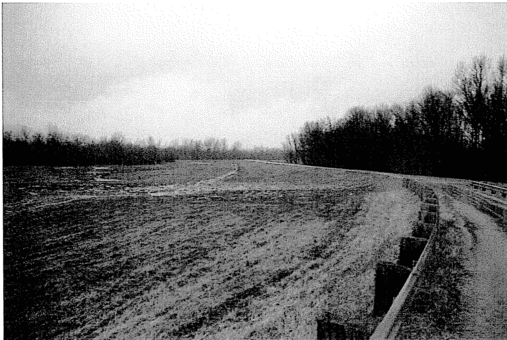
PHOTO 10 – PANORAMA FROM FLOOD WALL LOOKING EAST
