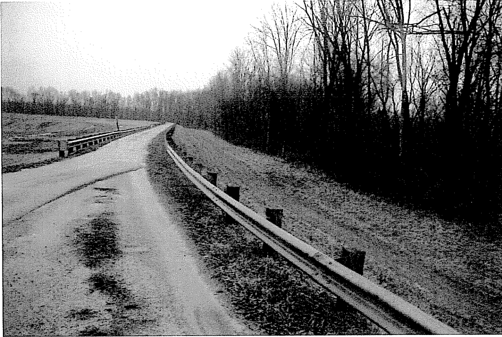
PHOTO 11 – PANORAMA FROM FLOOD WALL LOOKING EAST
